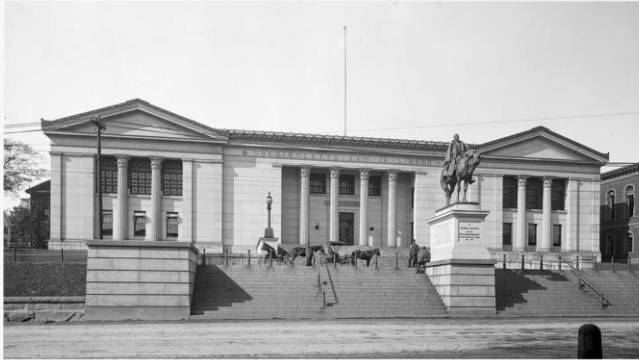
Courthouse Lofts. Worcester, Massachusetts
